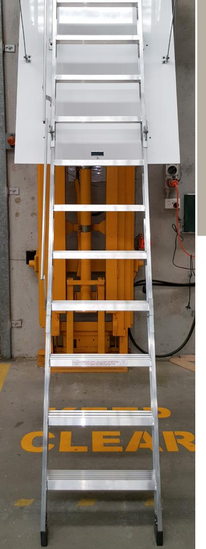
Pull-down access ladders are permanently fixed to the building and are thus safer and structurally more stable than freestanding ladders, removing any possibility of the ladder tilting, tipping or collapsing
